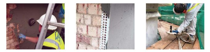
Homeshield in consultation with Wetherby Stone Products specified **Wethertex GRC backing coat render, a fibre re-enforced, high-polymer trowel applied render** which is designed to adhere well to difficult substrates and act as a water-proofing backing coat for subsequently applied decorative finishes. **Upvc angle corner/angle beads** were used to prevent the likelihood of any future corrosion.
